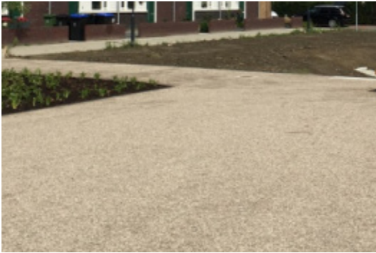
Paden halfverharding Ecodynamic Stabilizer Ijsselmix,
